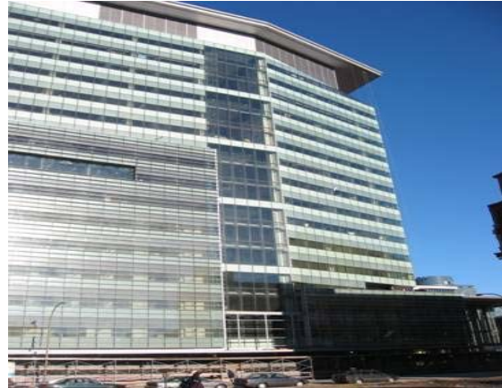
The new 16-storey building
