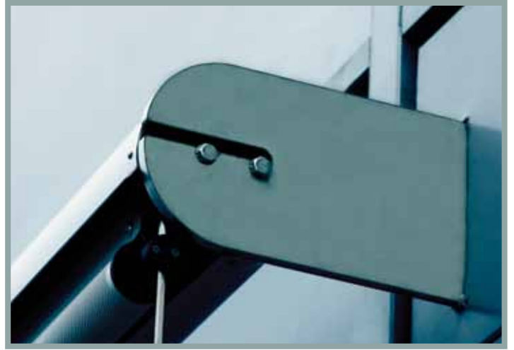
Seismic assembly with façade-integrated bracket
