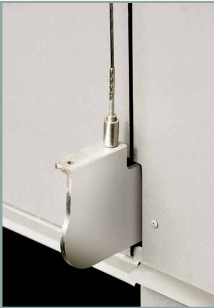
Customized, panel-integrated anchoring brackets
